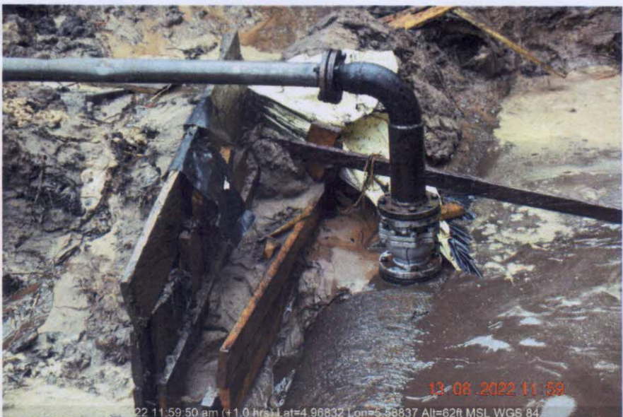
Fig. 3 The 4" Ball valve attached to the 24" for Oil Theft
